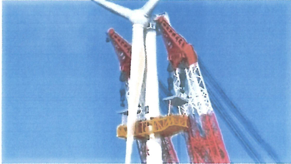
Fig. 5 A fully assembled Wind Turbine carried to its foundation offshore in China via ship.
