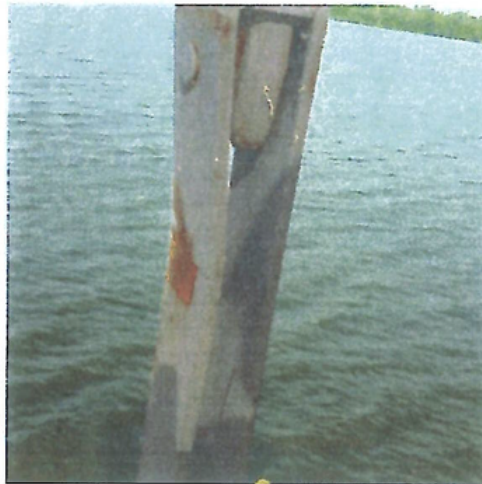
Fig.1 Bent structural gantry back stay – held during a load test!
